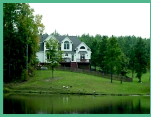
Example of a home lot with an RPA that was completely cleared and planted with grass. This is a violation of the county's Chesapeake Bay Preservation Ordinance.
