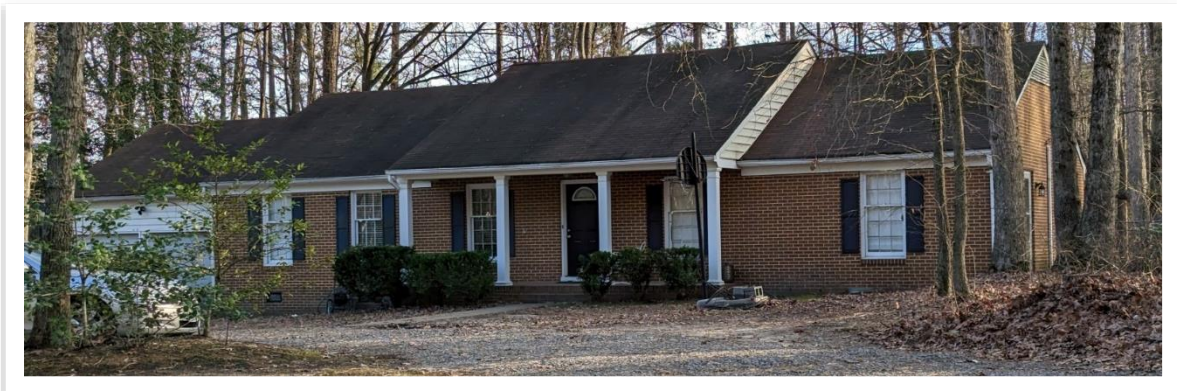
Figure 3 – Existing Site Conditions. View of the dwelling from Stigall Way.
