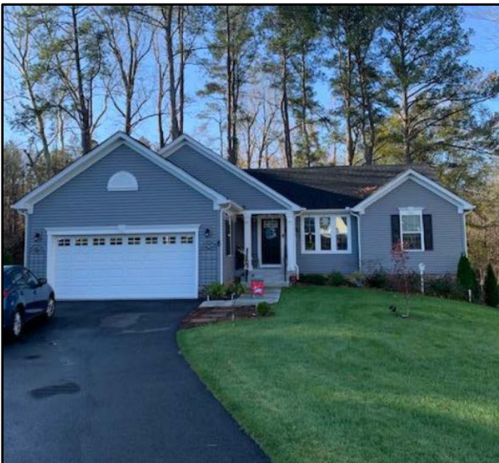
Figure 3 Existing Dwelling at 10331 Sandy Ridge Drive
