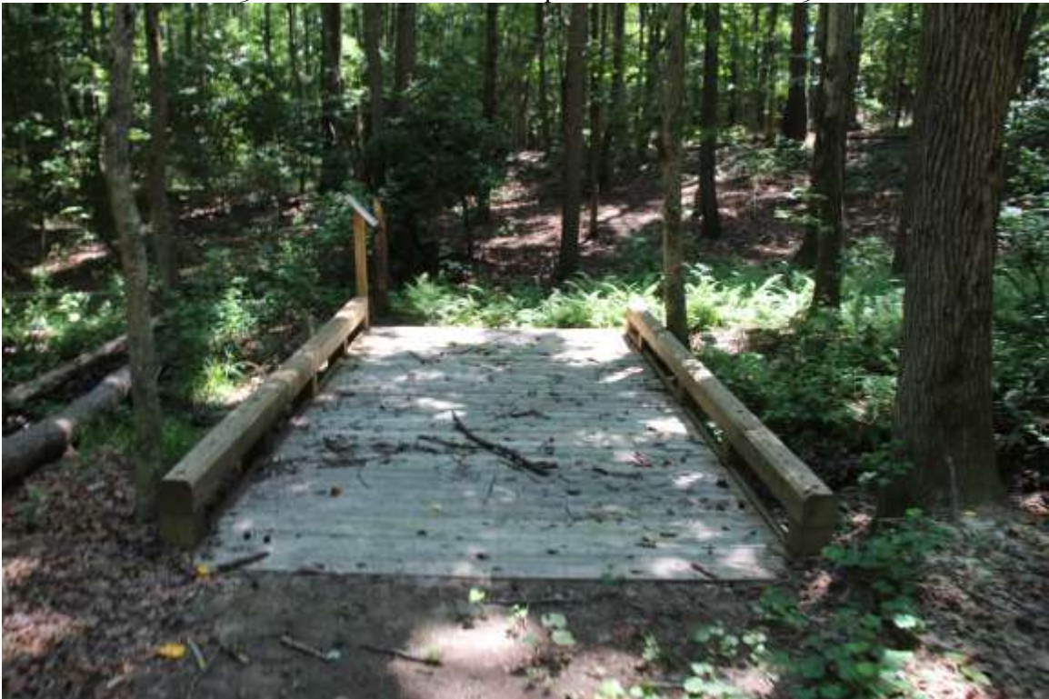
Photo 6. New footbridge, Walthall Baptist Church Tract, 6/19/2018.
