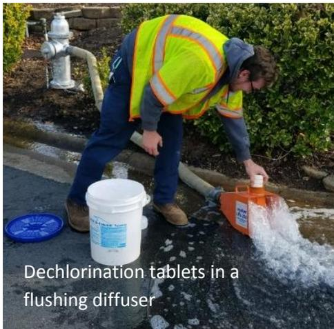
Dechlorination tablets in a flushing diffuser
