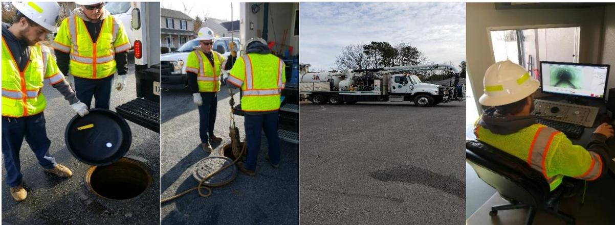
In FY18, 865 manhole dishes were installed, 179,503 feet of sanitary sewer lines were televised, 541,062 feet of sanitary sewer lines were cleaned and .28 million gallons per day of inflow and infiltration was reduced.
