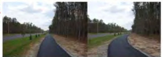
Completed 0.5 Mile Lake Margaret Home Owners Association Trail
