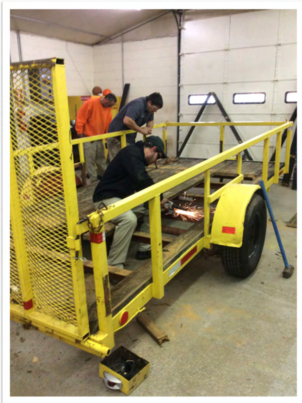
Replacing trailer decking with Brandon Ellis at Huguenot Park
