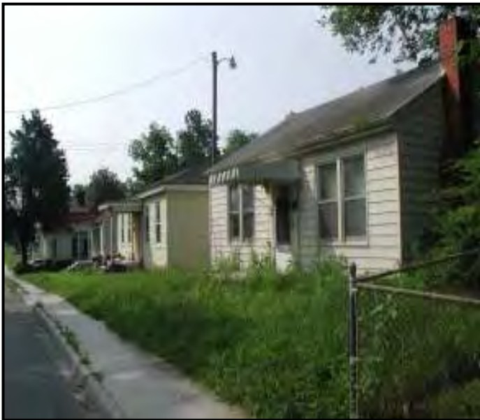
House Requiring Rehabilitation
