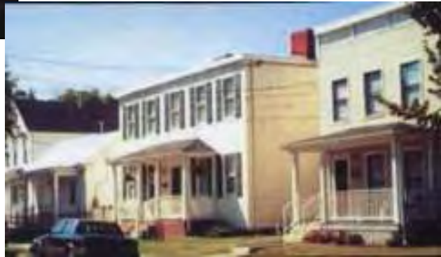
1600 Block of Decatur Street After Revitalization
